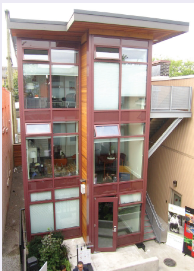
Atira's shipping container housing, Vancouver. © Atira.
